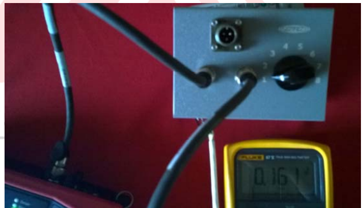
Figure 3— Testing the temperature circuit with a data collector and digital multi-meter on a DSB-MOD-08 Module.
