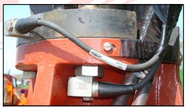
Axial and radial sensors installed on a pump- -Note the carefully routed cabling and the excellent protection of the cables within a few inches of where they exit the sensors.
