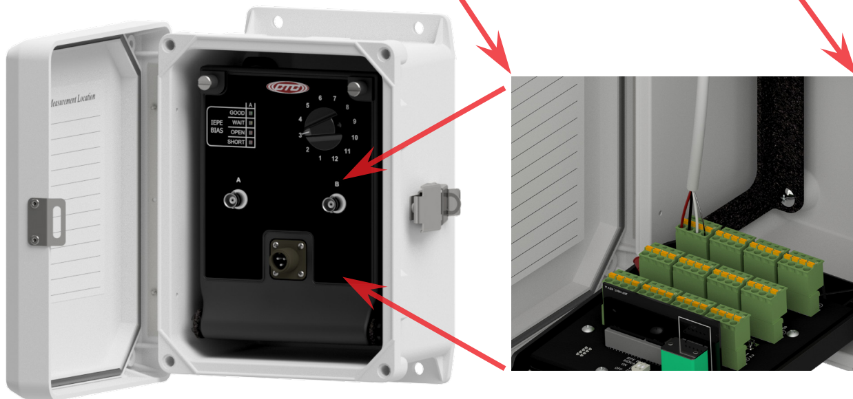
Figure 10. Field Wiring for 3-Conductor Sensor Inputs
