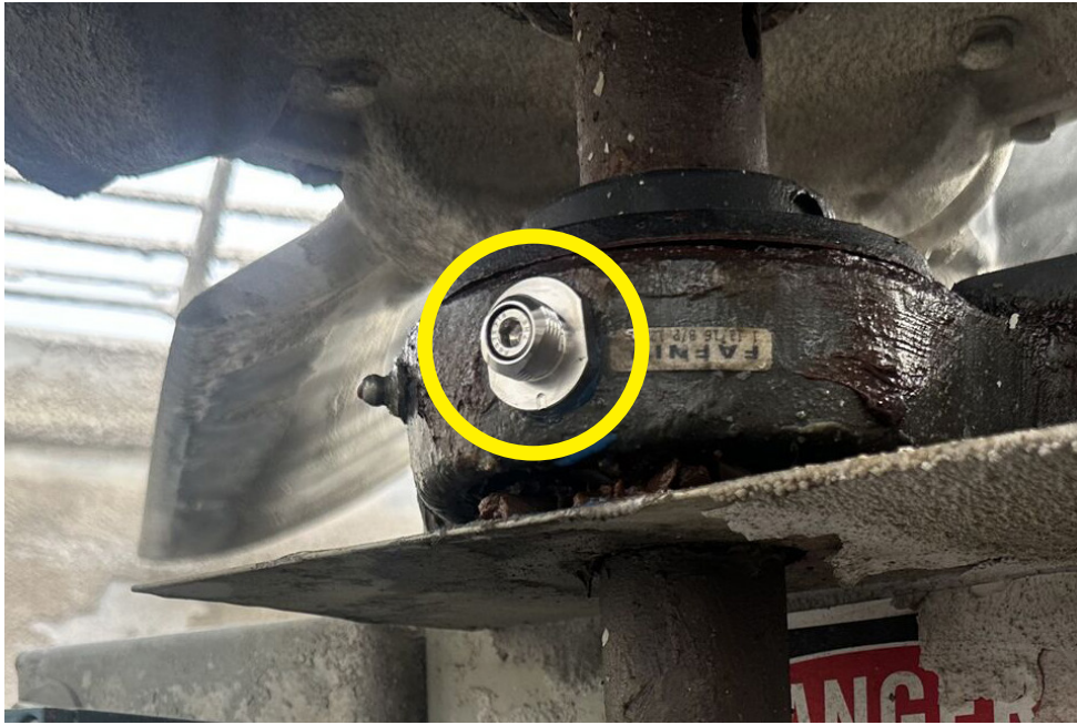
Fig. 4 Completed through-hole mount installation of an MH107-2B
