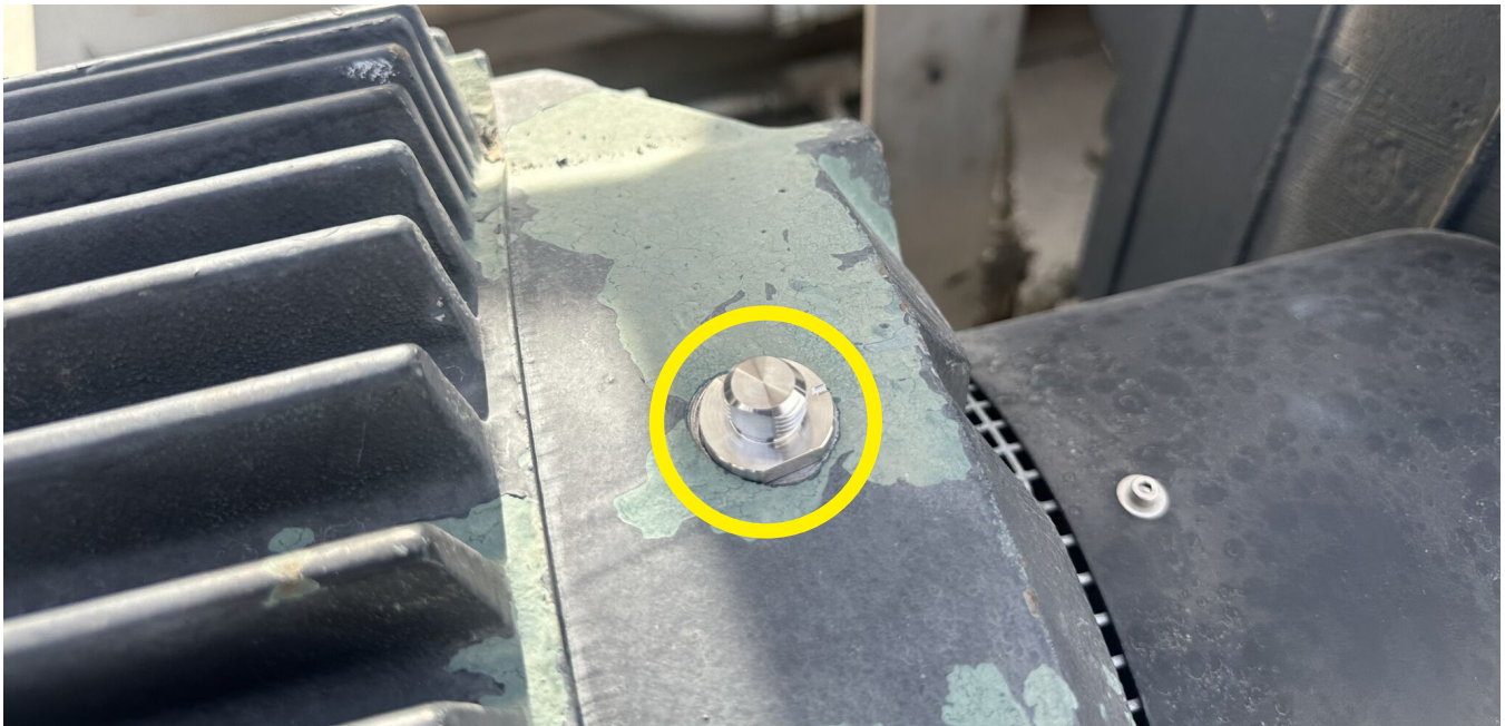
Fig. 3 Completed and cured adhesive installation of MH107-1B
