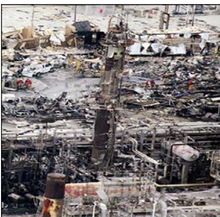
Figure 1— Hazardous ratings exist to help prevent explosions like this one.
