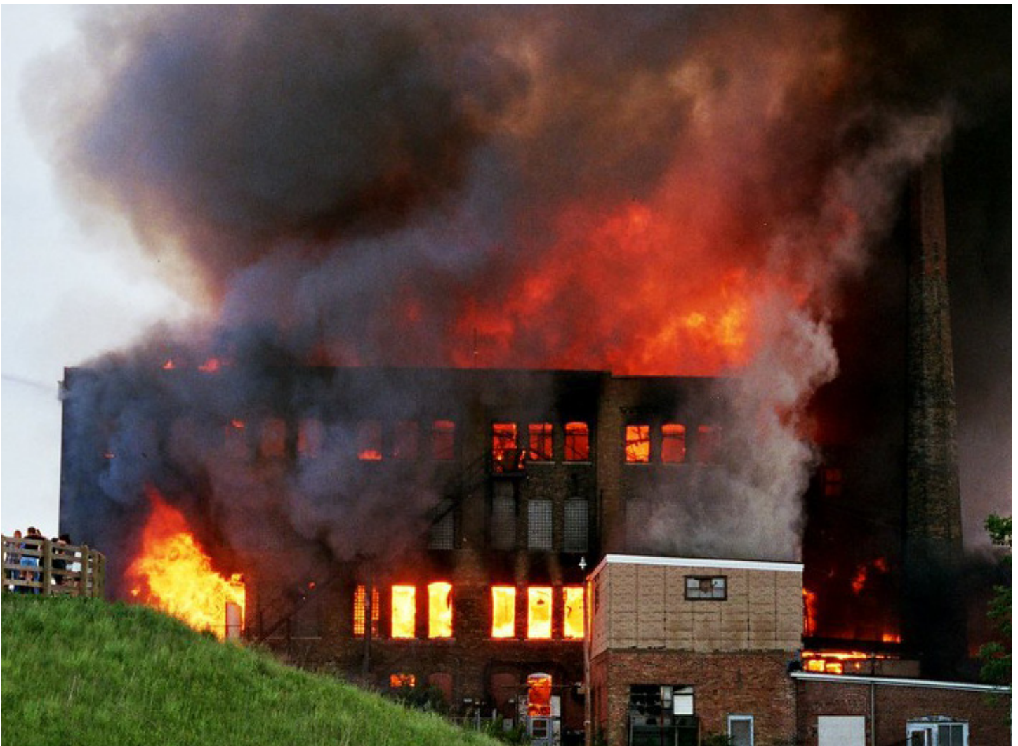
Hazardous ratings exist to help prevent catastrophic incidents like this one
