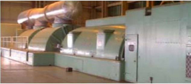
proximity probes are often used to monitor turbine shafts in power plants
